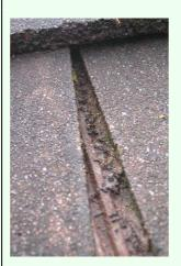
ISA members are reporting defects in relatively modern roofs (i.e. less than 30 years old) where the side interlocks between tiles become impeded by 'Fines' derived from the surface of the tiles combined with organic matter from moss - resulting in blockage and surface water spillage into the roof void, particularly on low-pitch roofs.
